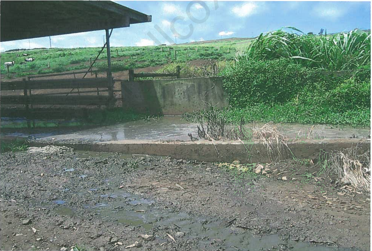
Photograph#7- This is another photo of the overflow spilling onto the dirt road.
