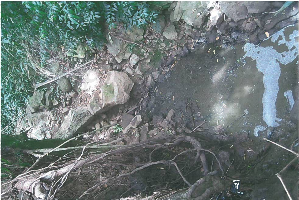
Photograph#13- This is photo of the brown sewage water entering the stream, with the stream bed above the enter point being dry.
